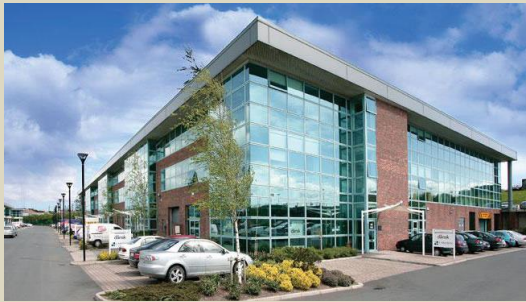
Promoting the development of new employment uses in the unincorporated parts of the county is a major goal of the 2035 General Plan.
