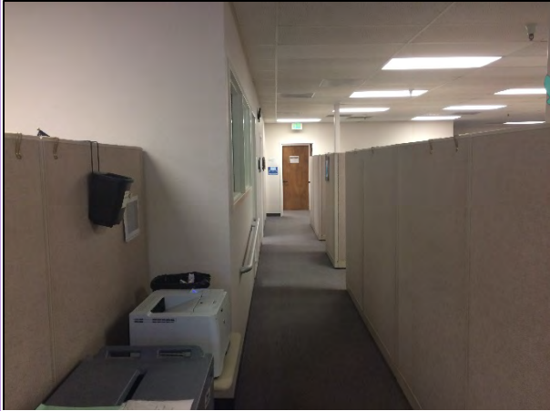
Hallway outside of Server Room
