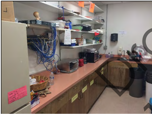
Work area, break room, IT closet
