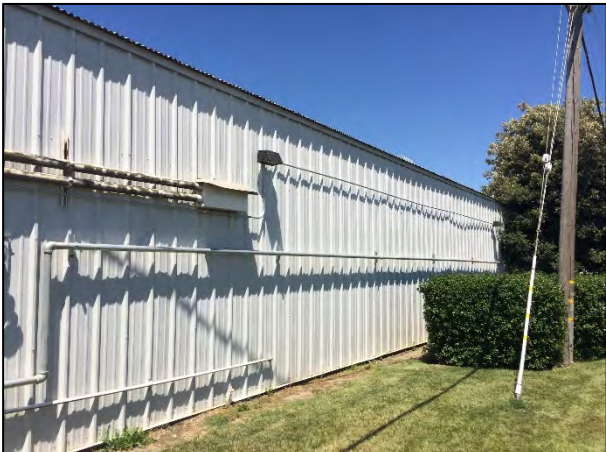
South Side of Building
