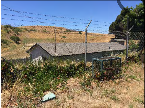
Exterior from Parking Lot
