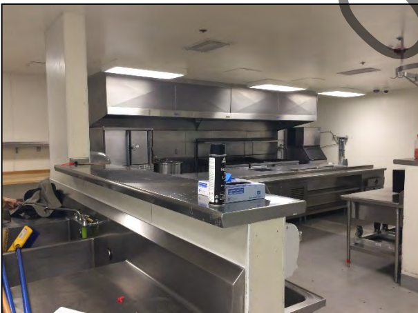
Kitchen under construction
