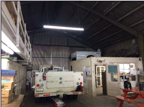
Truck Shop Interior
