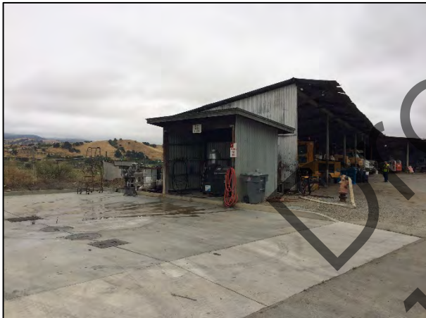
Vehicle Wash Area
