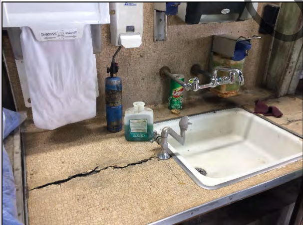
Truck Shop Interior
