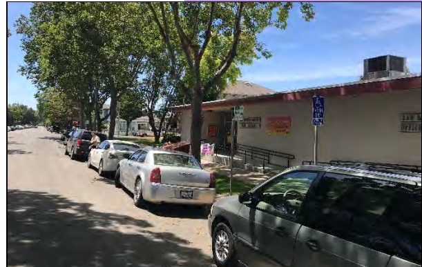
No. of Stories: 1 Square Feet: 15,570
