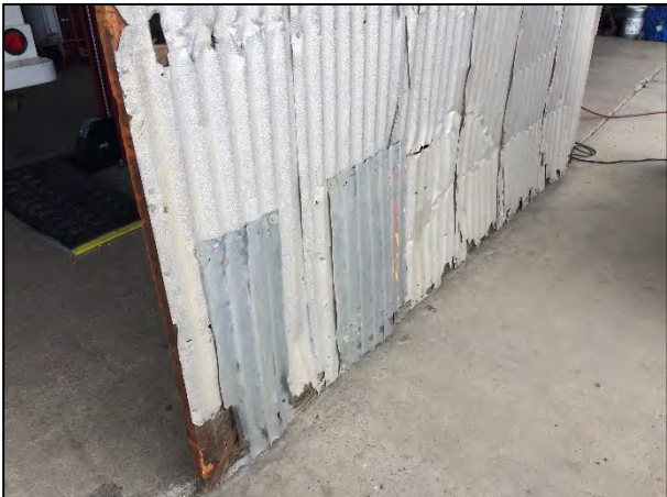
Truck Shop Exterior Siding
