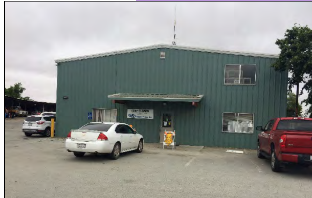
No. of Stories: 1 + Mezzanine Square Feet: 3,000
