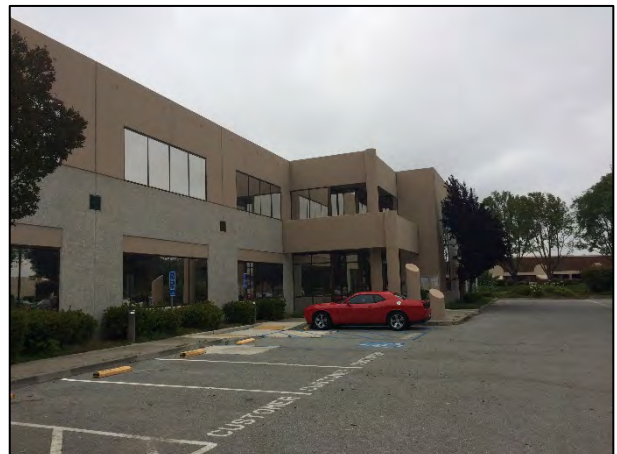
Front of Building
