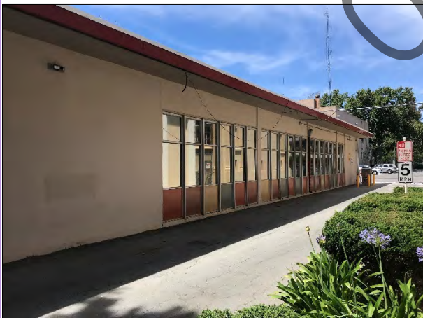
Exterior with outdated curtain wall system
