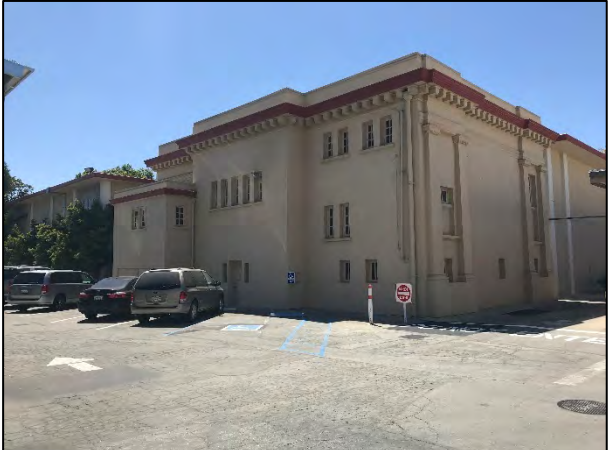
Exterior of Old Hall of Records
