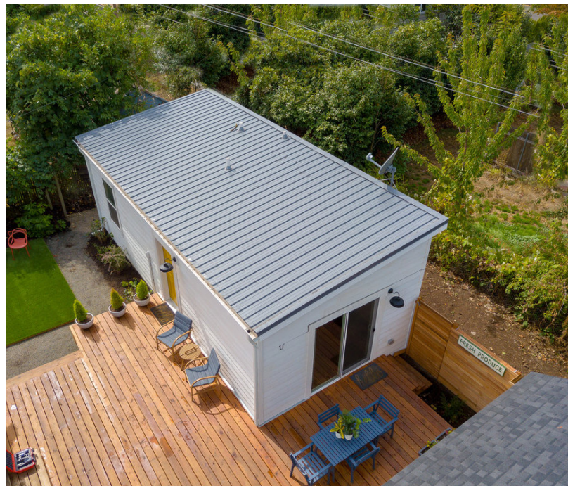
Above: Your ADUs placement on your property, heights, and window placement play a big role in keeping your neighborhood happy
