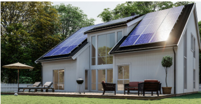
Above: Solar panels on the roof can help to generate power on-site while reducing long-term power costs
