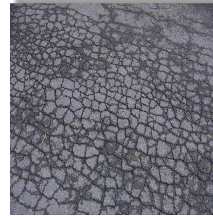
Alligator Cracking
