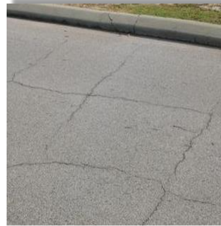
Block Cracking
