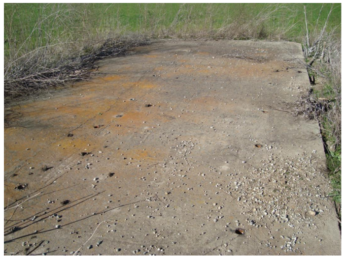
CONCRETE PAD LOCATED IN THE NORTHEASTERN AREA
