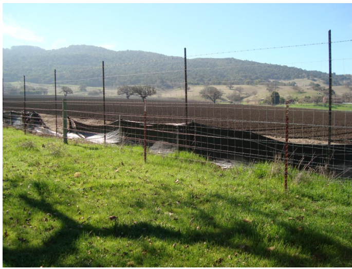
SILT FENCE ALONG WESTERN BOUND
