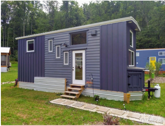
A Tiny Home with skirting installed
