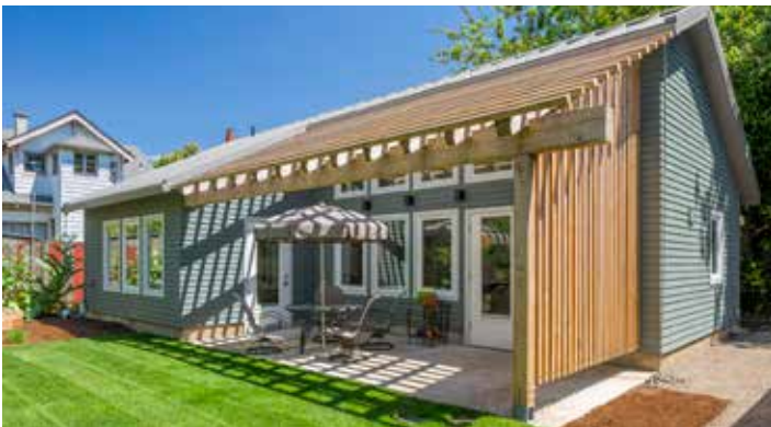
Above: Sustainable design enhancements can reduce your ADUs environmental impact (e.g. high efficiency building envelopes, FSC certified wood products, and low or zero VOC/ formaldehyde)
