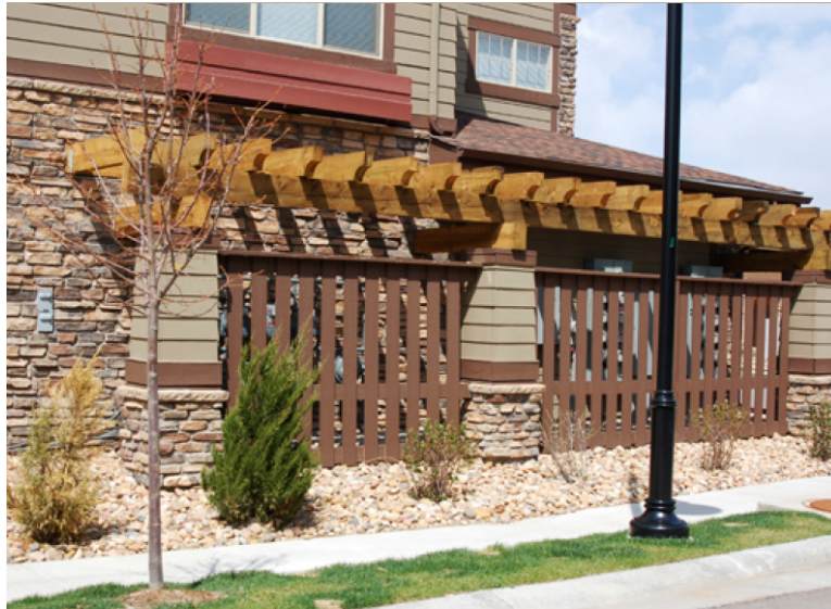
Screening of equipment (in this case, gas meters) is required.
