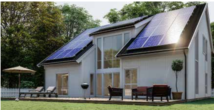
Above: Solar panels on the roof can help to generate power on-site while reducing long-term power costs
