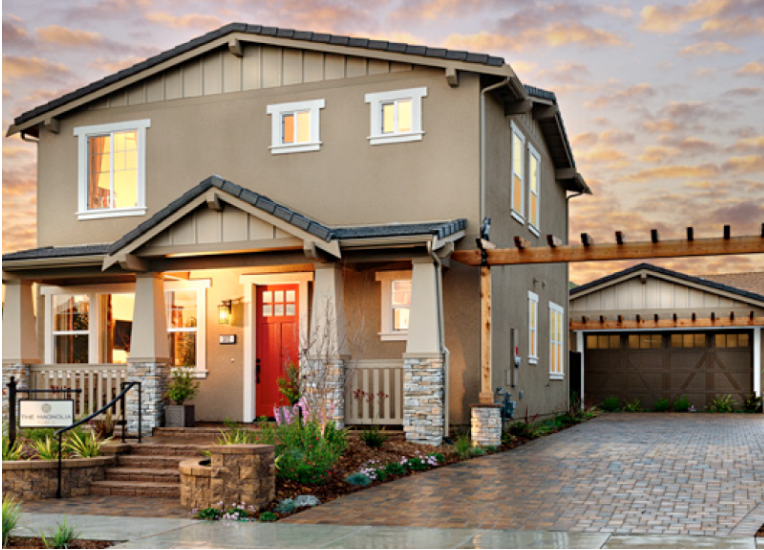
Example of a garage recessed from the front of the home.
