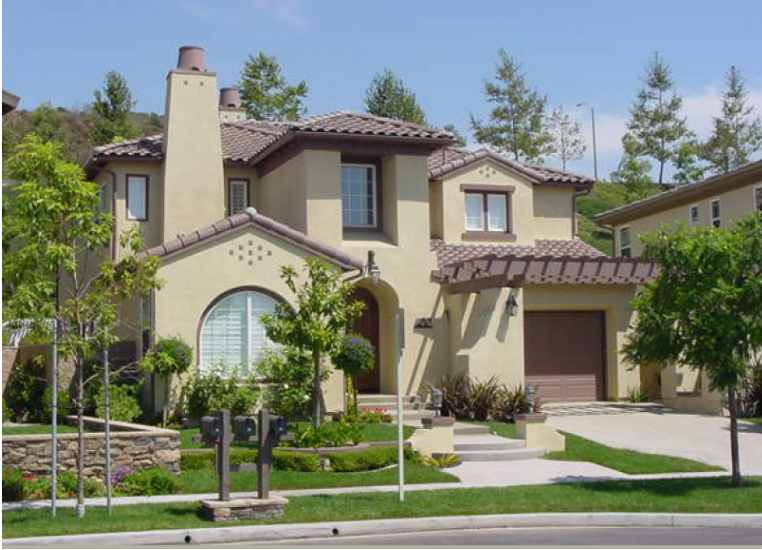
Example of the use of a variety of architectural features to reduce the “mass” of a single family home.
