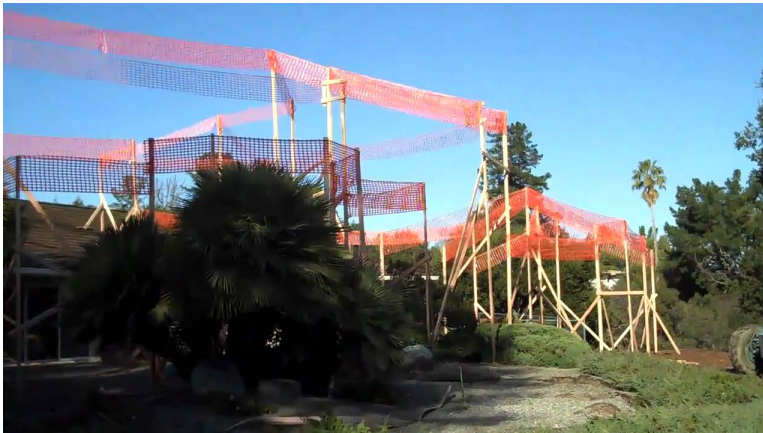
“Story poles” are used to show the general outlines of a proposed structure.
