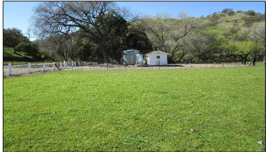
On parcel 0271500030, looking southwest toward the pump house and Project site.
