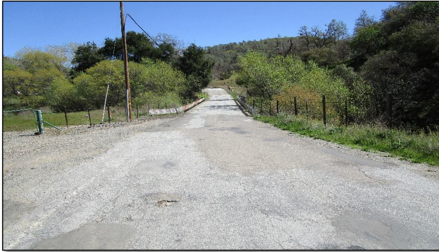
On Panoche Road, looking east toward the Project site.
