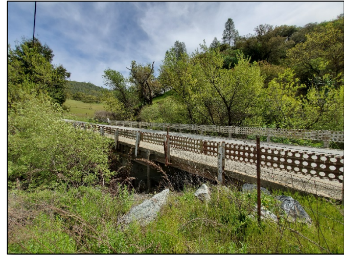
Panoche Road Bridge looking southeast.
