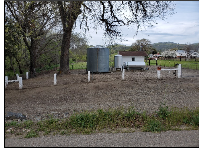
Spring box and pump house north of Panoche Road, east of Tres Pinos Creek, looking northeast.
